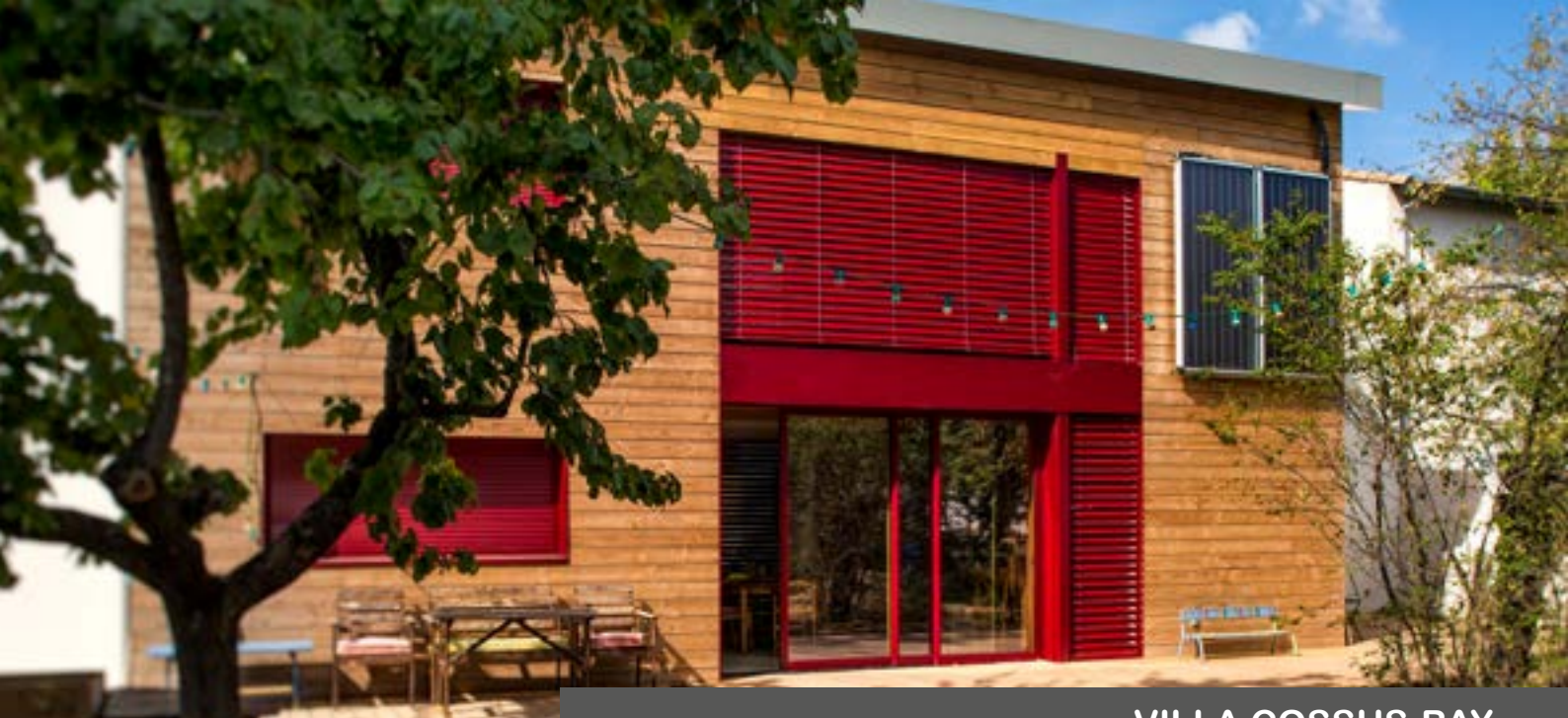
Photo © Mathieu Bay | Architecte : Lhenry Architecture
